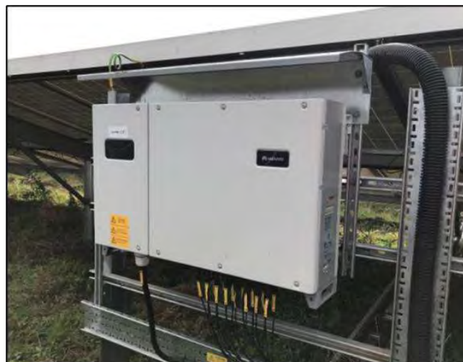
Figure 2-1: Typical String Inverter
